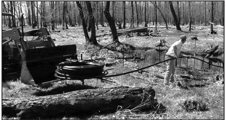
Laying large rolls of pipe can be a daunting task. Here a spinning jenny is used to make the job easier.
